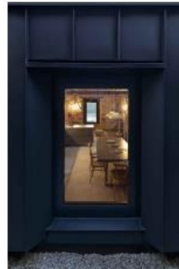
'Greencoat PLX' metal cladding
